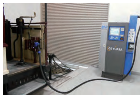
急速充電風景 Rapid charging
